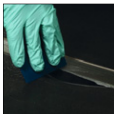
10. Smooth the compound immediately and let it cure for about 60 minutes.
