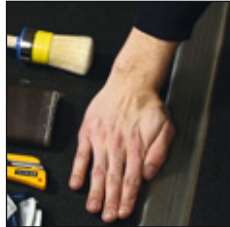
2. Make sure the damaged area is smaller than your hand (max. 100 cm 2 ).
